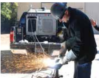
Handheld cutting in the field
